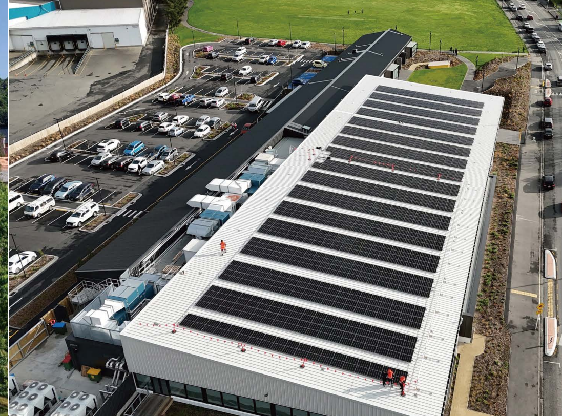
Metal Roof Mount-New Zealand
