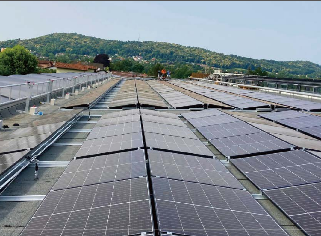
East & West Ballasted PRO-Switzerland
